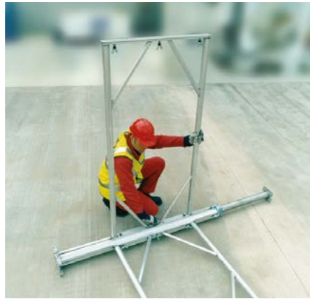
2. Connect ledger frame vertically to leg
