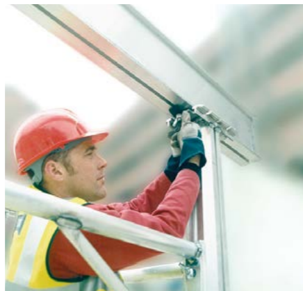
8. Fix primary beam to headplate by means of two TITAN clamps
