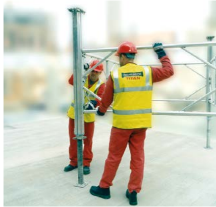
5. Connect both sides to form a four leg tower
