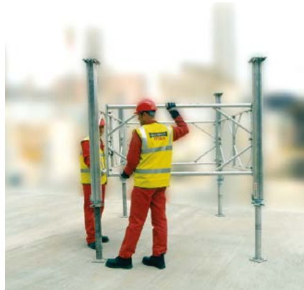
4. Repeat 1 to form 4th side of bay and then lift both sides of bay into position
