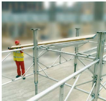
7. Place intermediate transoms and scaffold boards or walkway platforms and handrail frames in position for fixing of TITAN aluminium beams
