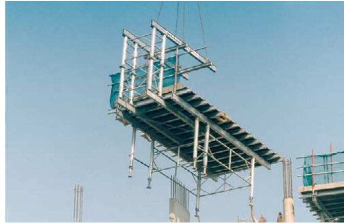
'C' Hook for removal of small edge tables up to 1.0 tonne assembled from standard TITAN components
