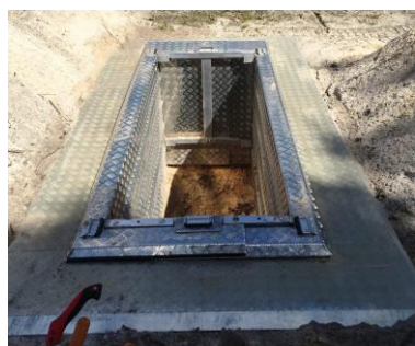
Multi- Cultural shoring in use
