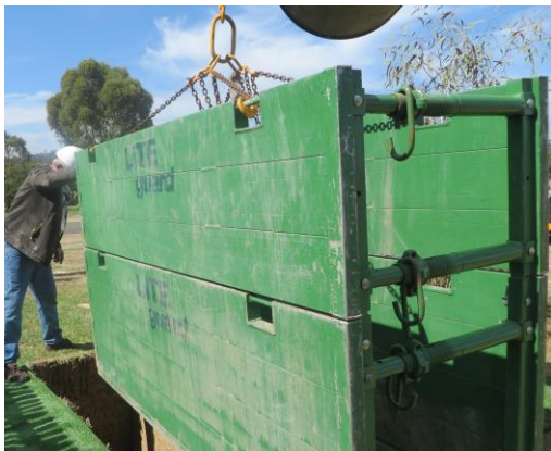
Installation of the shields
