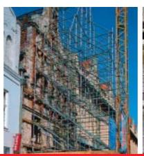
The **building industry** is presenting high demands for load-bearing capacity and versatility in scaffolding. Allround scaffolding sets the standards: one system, as **bricklayer's scaffolding, work scaffolding, support scaffolding** or **inspection scaffolding** – supporting loads of up to 6 kN/m².
