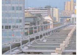
With Layher Allround equipment you can easily build **cage protection** for flat roofs and surfaces in accordance with German VBG 37 regulations for building work: without improvisation and without wasting time, a quick solution is always possible; a few additional parts (such as guard rail uprights, stiffeners for the uprights, a ballast tube and ballast) are added to the available standard material.
