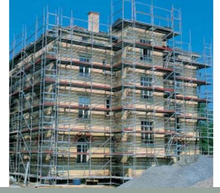
Layher Allround equipment as a **bricklayer's scaffolding**, either 1 m or 1.4 m wide: to lay blocks or bricks from scaffolding, you always need just the right platform height. With Layher Allround equipment, you can raise the working levels in 50 cm or 100 cm steps.
