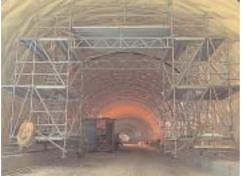
Layher Allround equipment as **rolling tower** and **birdcage scaffolding:** the flexibility of Allround's dimensions makes particularly material-saving solutions possible – thus adapting to the space available and at the same time supporting the required loads.
