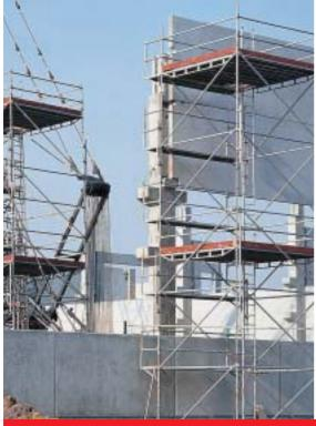
Bracing to the centre of the joint and wobble-free wedge-head connection ensure extremely rigid structures that can also be quickly positioned as pre-assembled scaffolding units using a crane.
