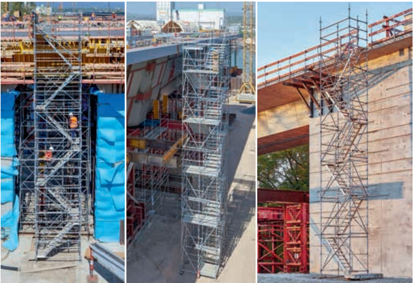
Top: Construction stairway tower integrated into the birdcage scaffolding as the main access and escape route and at the bridge construction site. Bottom: Individual and independent stairway towers (Allround modular stairway tower and construction stairway tower 200).
