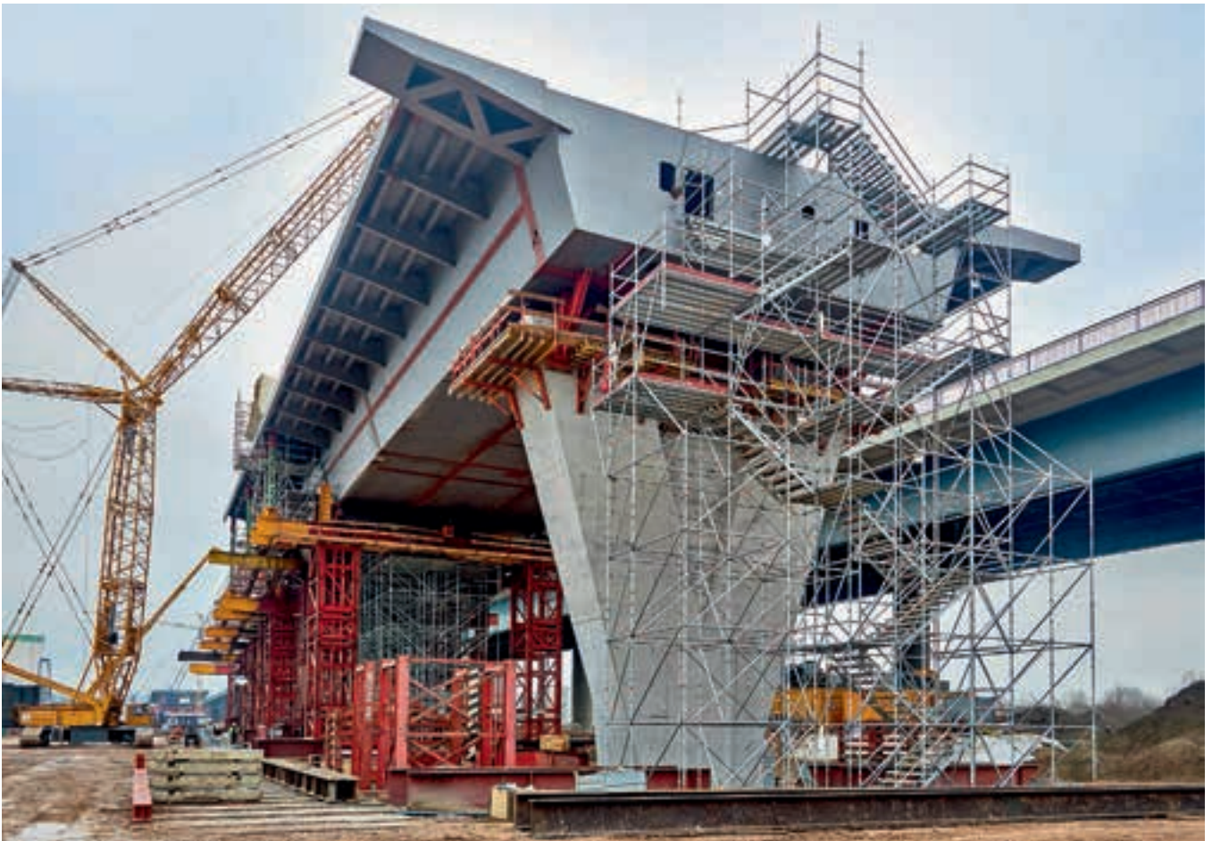
Top: Construction stairway tower integrated into the birdcage scaffolding as the main access and escape route and at the bridge construction site. Bottom: Individual and independent stairway towers (Allround modular stairway tower and construction stairway tower 200).
